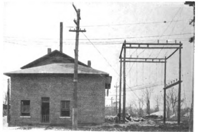
PROSPECT SUB-STATION, COLUMBUS, DELAWARE & MARION
