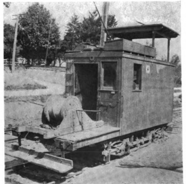
CAR FOR STRINGING WIRE, COLUMBUS, DELAWARE & MARION
