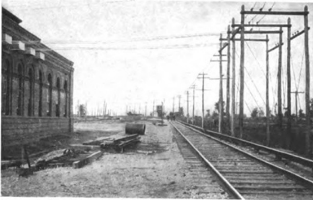
LINE ANCHORAGE AT POWER STATION, SCIOTO VALLEY
