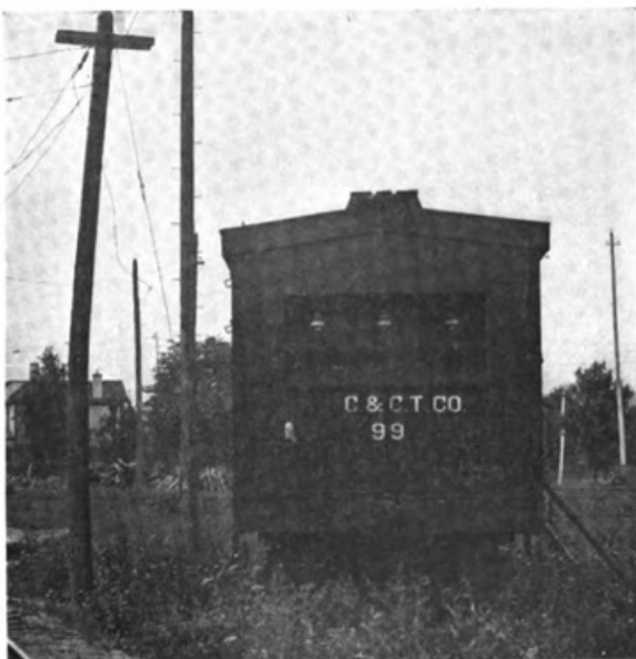
PORTABLE SUB-STATION, CINCINNATI & COLUMBUS
