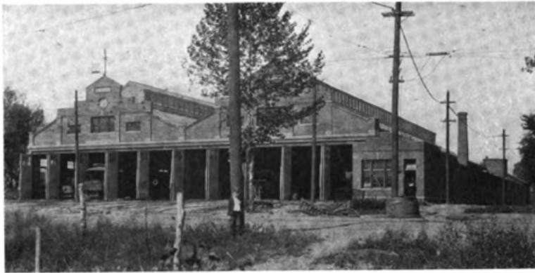
CAR HOUSE AND SHOPS AT NEWARK, OHIO, COLUMBUS, NEWARK & ZANESVILLE
